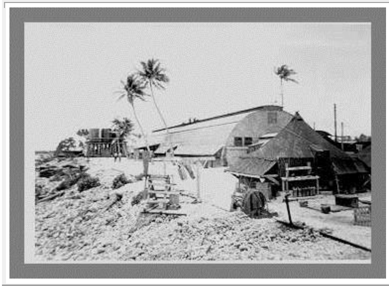
The rear of the mess hall located on the North or ocean-side of the islet. The large wooden tanks in the far rear were where sea water was converted to fresh water. Photo © 2001-9
